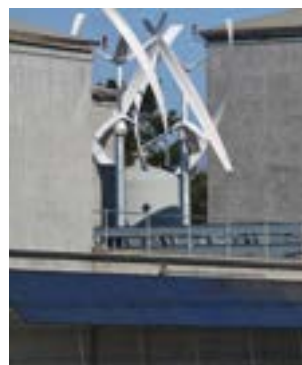
SES Hybrid solar and helical axis turbine wind power system for US Navy R&D.
