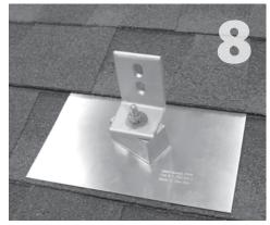
Using the rack kit hardware, secure the racking (L-foot) to the mount using torque specs from racking manufacturer. If racking manufacturer does not specify torque setting, tighten to 13 ft.-lbs.
