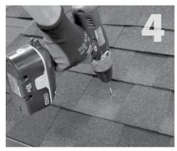
Using drill with 7/32" bit, drill pilot hole into roof and rafter, taking care to drill square to the roof. Do not use mount as a drill guide. Drill should be 'long style bit', aka 'aircraft extension bit' to drill a 3" deep hole into rafter.
