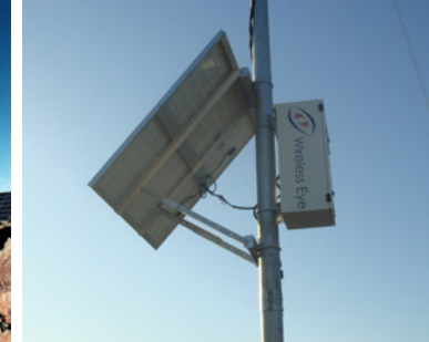
Wireless security camera mobile trailer
