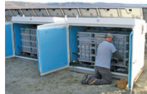
Large battery enclosures for MAPPS solar powered air monitoring system.
