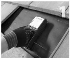
Remove the tile at selected location of the mount. Locate and mark the center of the rafter.
