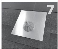
Install flashing over mount.
