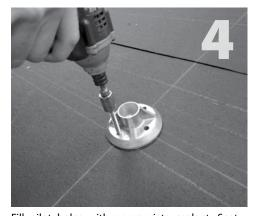
Fill pilot holes with appropriate sealant. Seat grade 8 bolt through bottom of QBase. Place QBase over drilled holes and secure lags in place, to a solid, snug fit.
