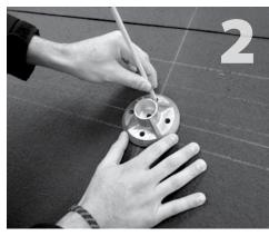
and horizontal holes over snapped line. Mark holes for drilling.
