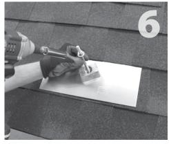
Slide mount (item 1) back into position. Prepare hanger bolt (item 3) with 1 hex nut (item 5) and 1 sealing washer (item 4), insert through block into hole and drive hanger bolt into rafter, tightening to a solid snug fit. \*
