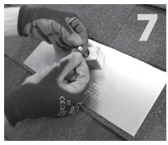
Insert EPDM rubber washer (item 6) over hanger bolt into block.
