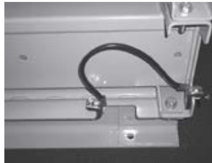
Figure 3: Cable Assembly Installation
