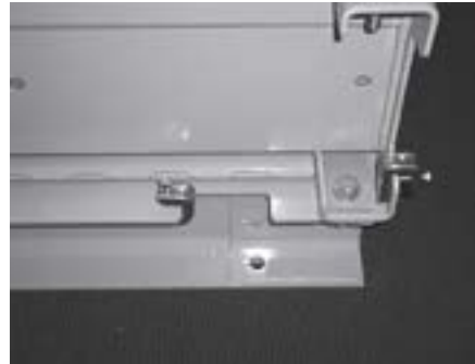
Figure 1: Beam Clamp Installation
