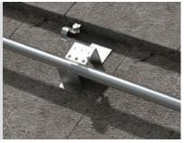
4 Use self-tapper screws or included hardware to mount conduit straps or junction box bracket. Refer to the NEC for required conduit spacing.
