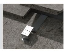
**3**Lower lifted tile and adjust adjacent tiles if any tile spacing has been disturbed by the installation.
