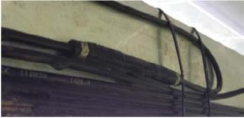
Fig. 9: Fastening of the connector tight to the mounting structure can cause moisture build up between connector and rail, damaging the connection
