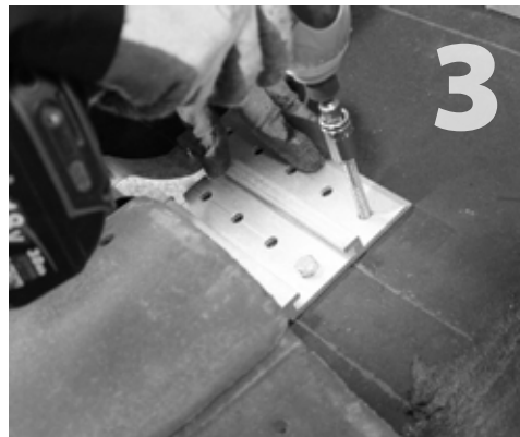
3 Connect hook (item 3) to base plate and drive lag screws (item 2) into rafter through the two holes to a solid, snug fit. DO NOT over tighten lag screws, this may compromise their holding strength.
