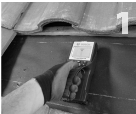
1 Remove the tile at selected location of the mount. Locate and mark the center of the rafter.
